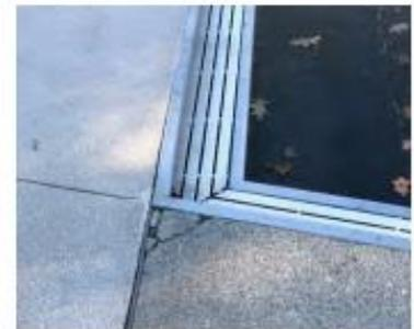
*Figure K: Pool Deck Cracking*
