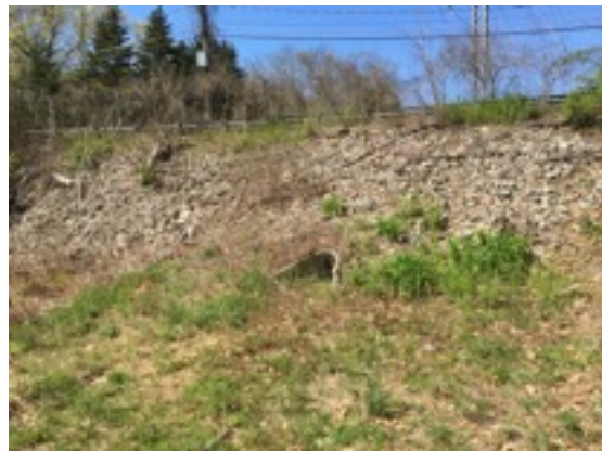
"Conant Road bridge: filled in 1980s"
