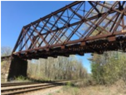
"Existing Bridge Over MBTA Fitchburg Commuter Rail."
